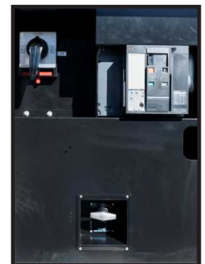
3 position voltage selector switch & parallel
