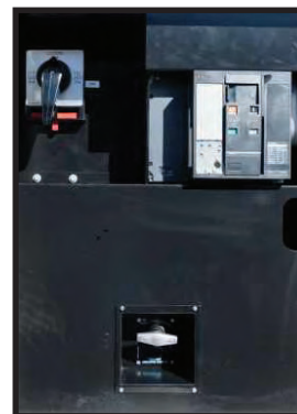
3 position voltage selector switch & parallel
