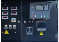
Deep Sea 8610 amps Parallel Controller. Digital amps gauges for quick reference.
