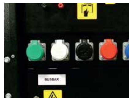
Multiple camlocks are standard in all models.
